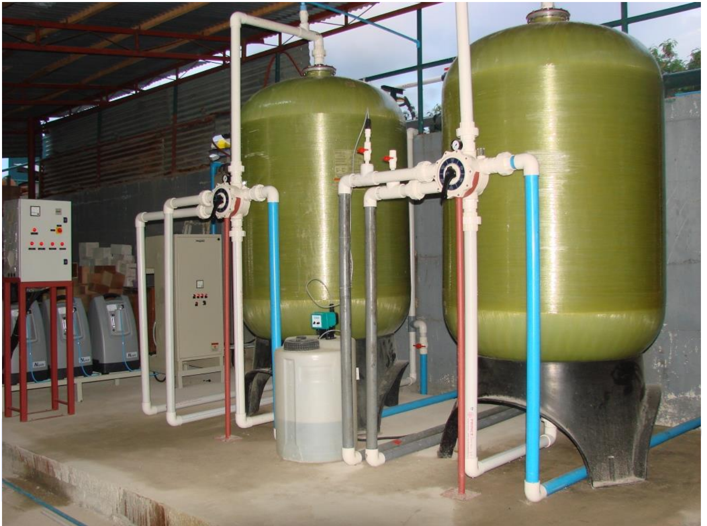
Fig. 2, Tertiary Treatment: Charged Activated Pressure Filtration + Online Ozonation
